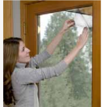
Homeowner installation of low-e interior surface film.
