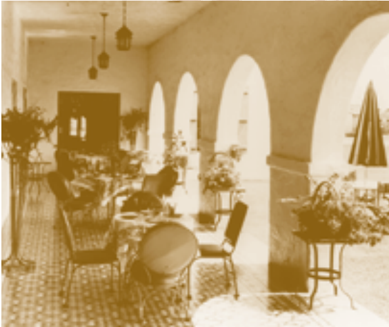
SOUTH PORCH OF OFFICER'S CLUB, GRAND CENTRAL AIR TERMINAL GLENDALE, CA 1933
